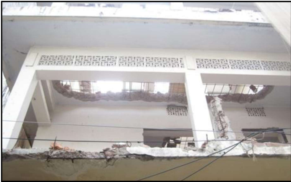
Fig. 3.2 Building under Demolition
